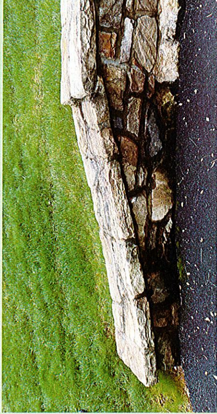
Existing Tapered Wall
