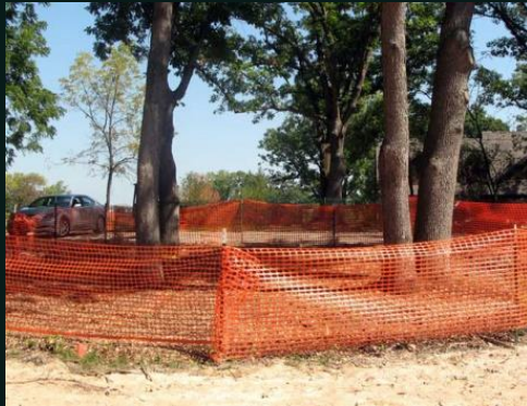
Tree Protection During Construction
