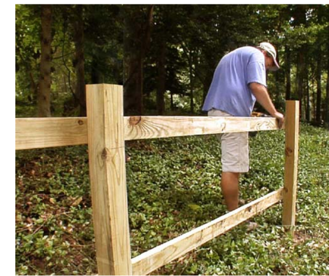
TEMPORARY WOOD TREE PROTECTION FENCE WITH TWO RAILS (ALL WOOD MAY BE UNTREATED, 2x4 SIZE OR LARGER)
