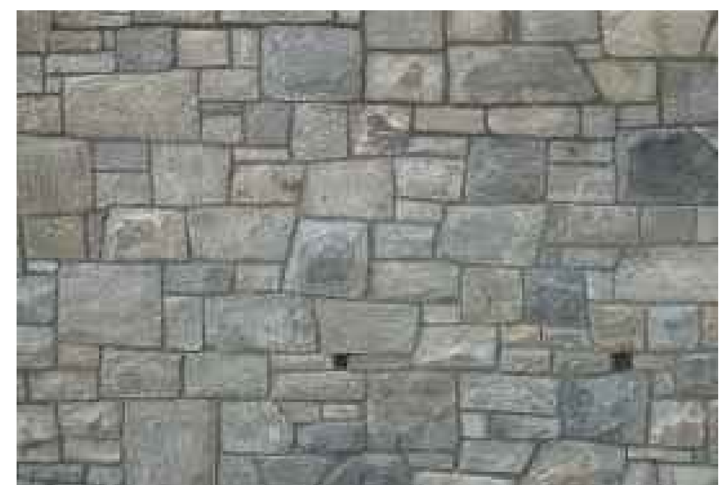
STONE VENEER RETAINING WALL
