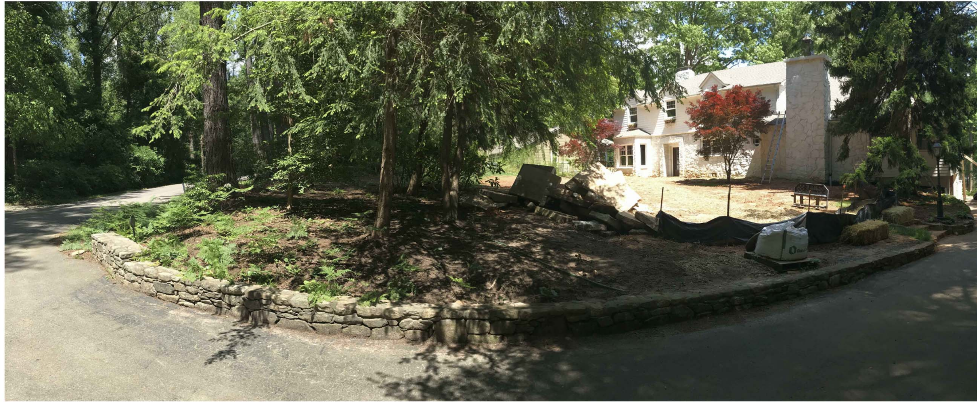
EXISTING RETAINING WALL AT FOREST ROAD
